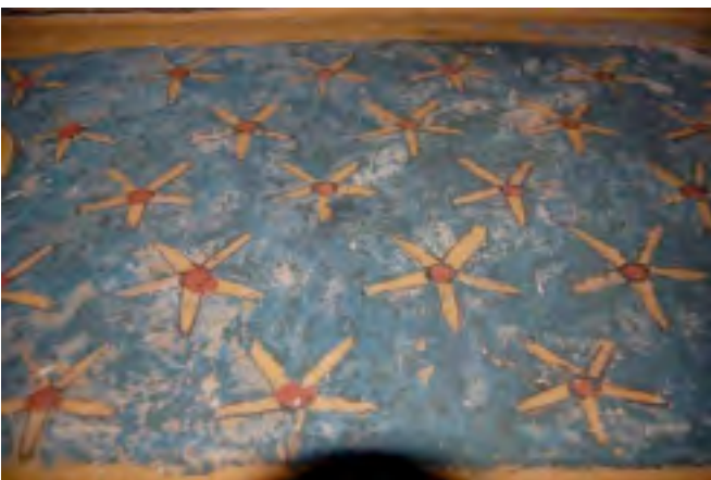
Stars painted on TT223 ceiling (Photo: SCA)
